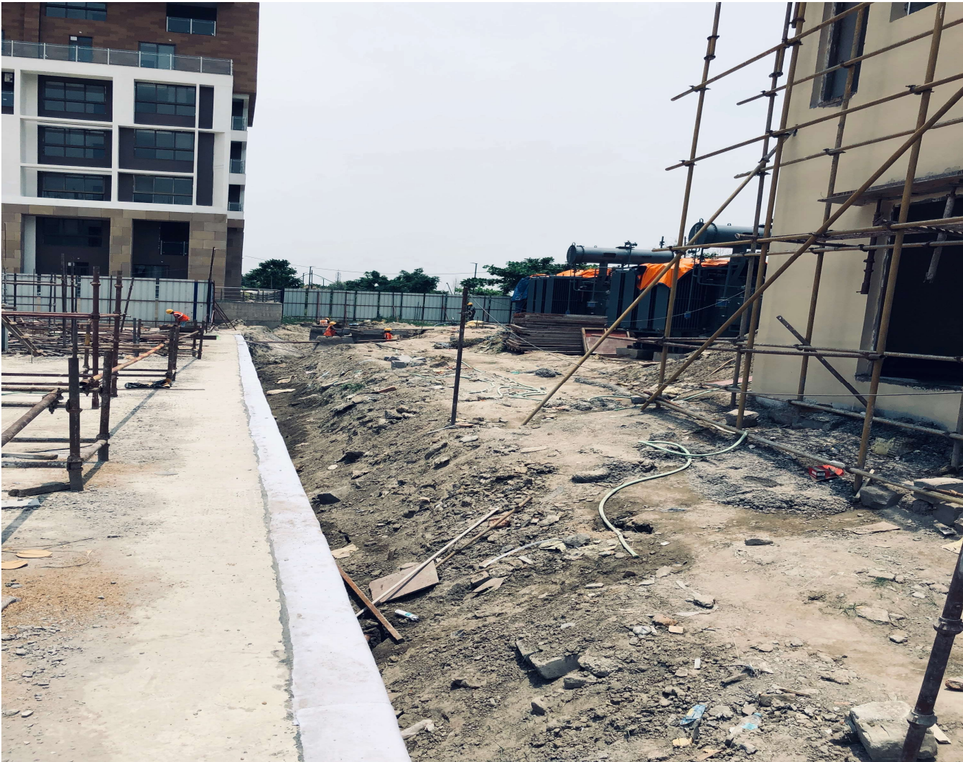
INFRASTRUCTURE WORK: Service Pipe laying started
